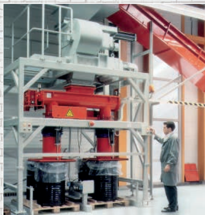
Recycling plant for sodium-vapour lamps
