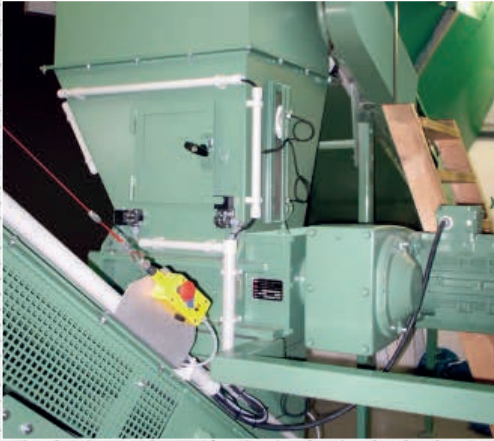
Wastepaper-shredder under a dropping chute in an administrative building
